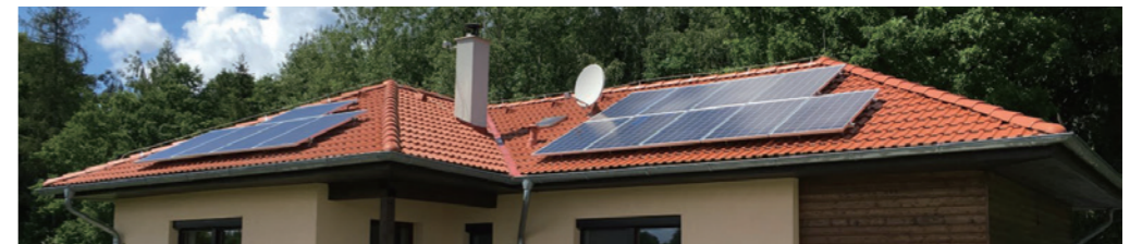
ENERGY STORAGE SYSTEM
